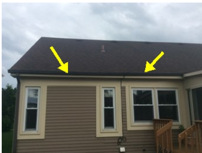
Gutters are sagging and need repair.
