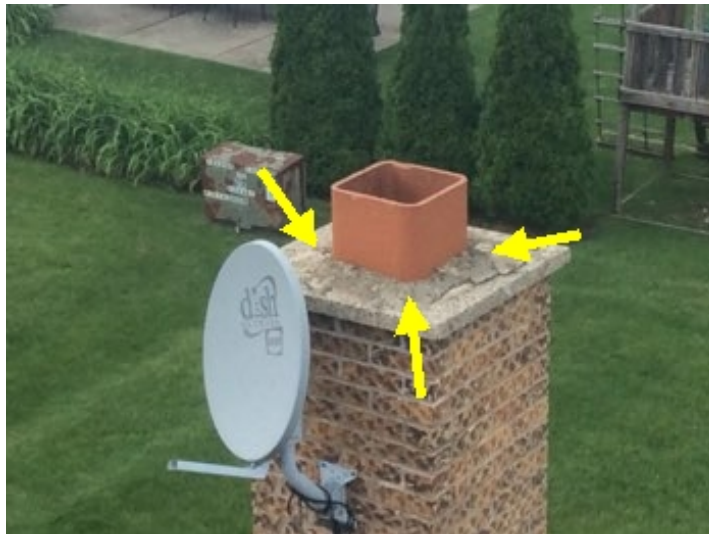
Evidence of cracks in masonry chimney cap.
