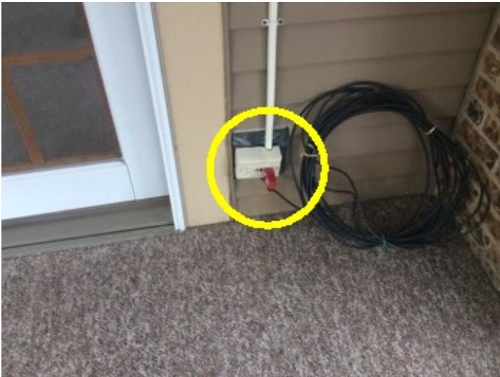
Defective GFCI at rear exterior outlet.
