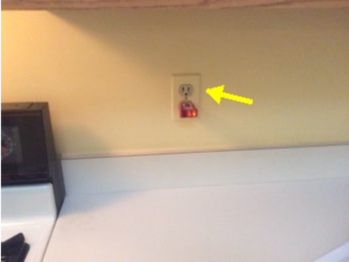
Recommend installing GFCI's on kitchen countertops where missing.
