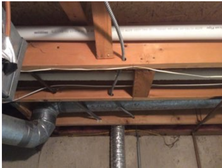
Improper holes bored through joists.
