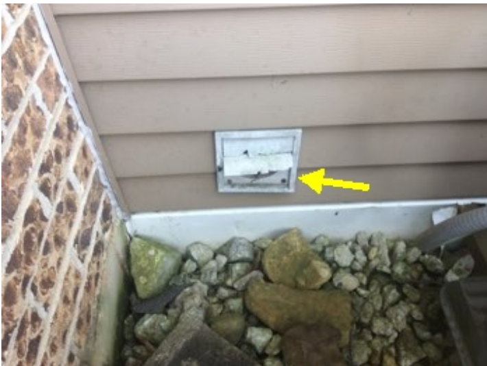
Damaged vanes on vent jack need repair.
