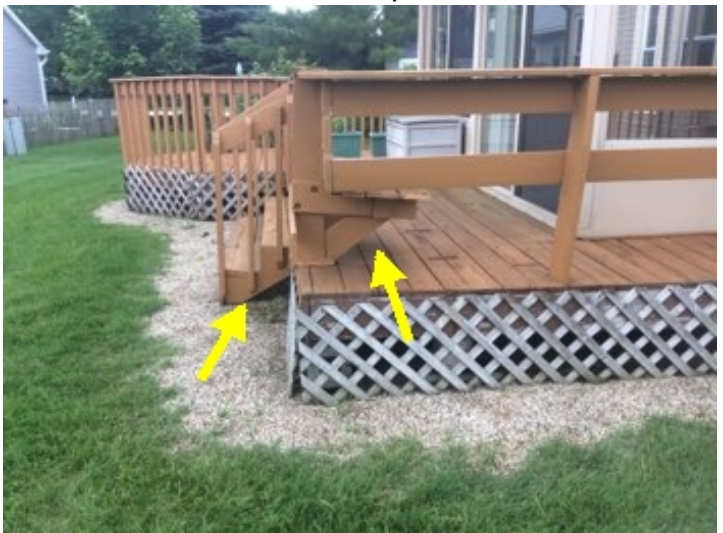
Unevenness of deck indicates the possibility of frost heaving.
