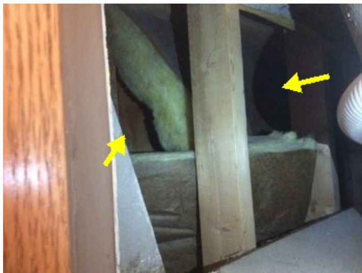
Missing insulation on outside wall under whirlpool tub.
