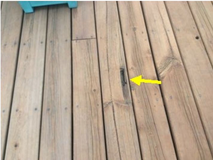
Evidence of wood deterioration observed.
