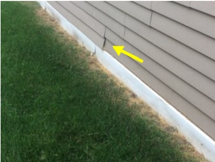
Loose and damaged siding should be repaired.
