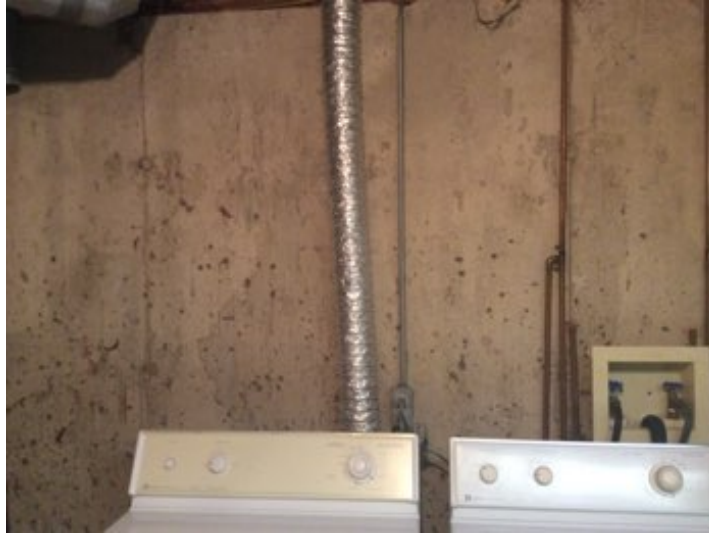
Recommend solid walled metal pipe for dryer vent.
