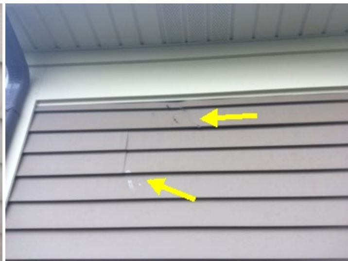
Damage to siding visible.
