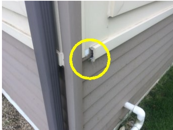
Recommend to repair or replace damaged trim.
