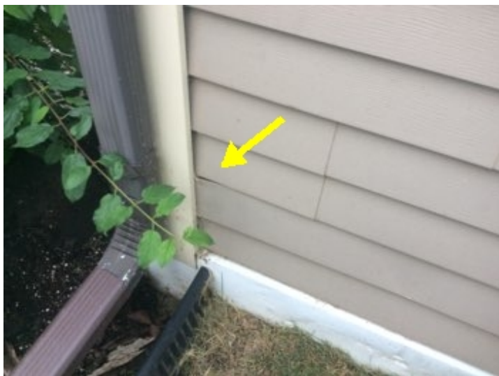
Evidence of cracks in siding present.
