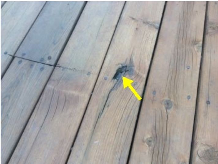
Evidence of wood deterioration observed.
