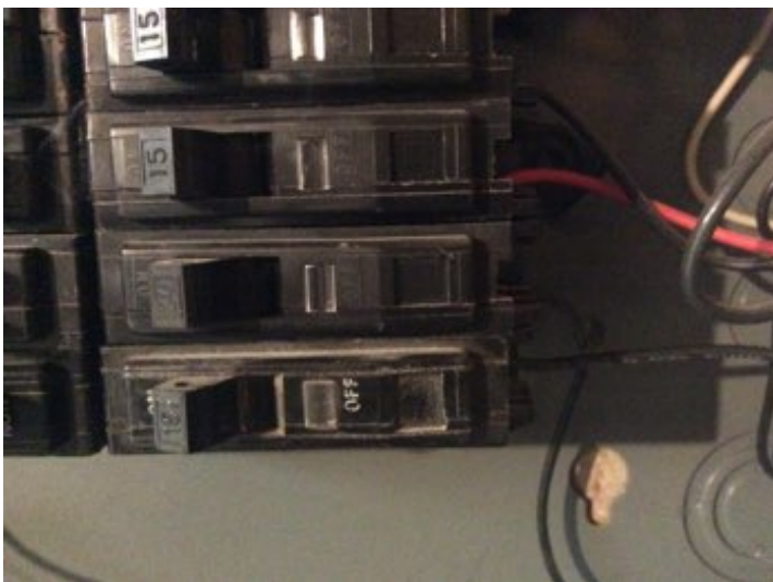
Overfusing at circuit disconnect observed.
