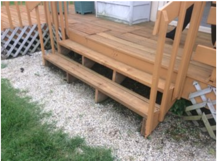
Deck does not appear to properly supported and needs repair.
