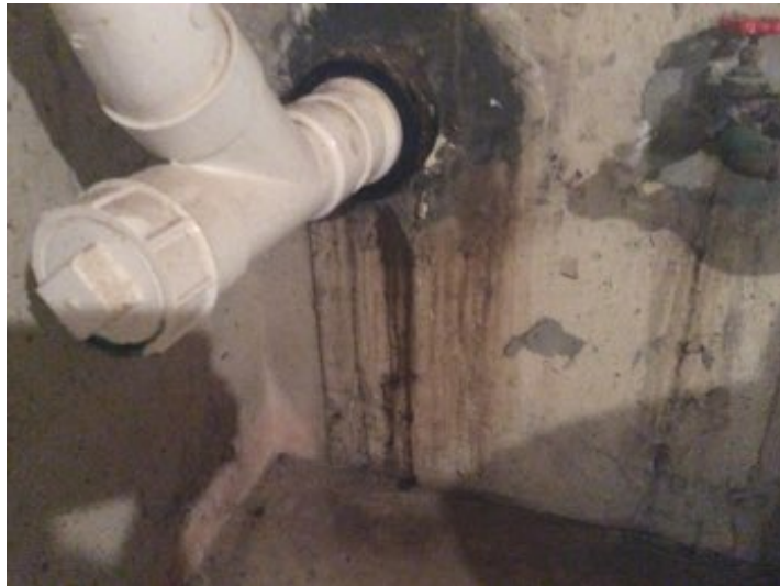
Evidence of seepage stains on foundation wall.
