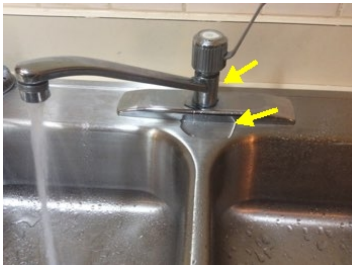
Faucet is leaking and needs repair. Possible cartridge or O-Ring.
