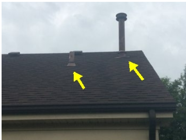
Exhaust vent pipe flashing has lifted and needs repair.
