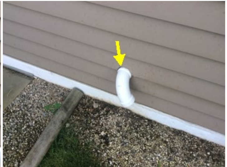
Recommend caulking at open seams.
