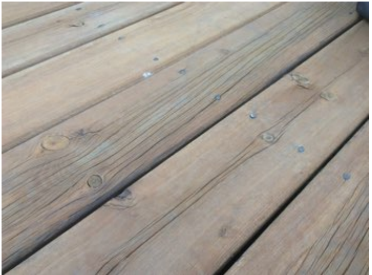
Evidence of nails/screws popping on the deck boards.
