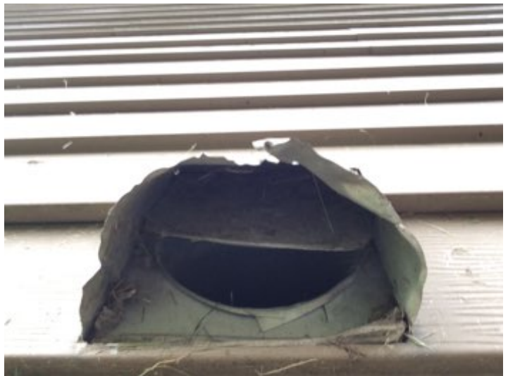
Damaged vent jack needs repair.
