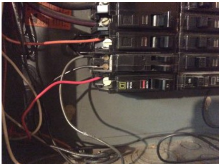
Tandem or mini breaker has been installed in service panel.
