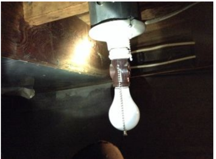
Porcelain light fixture is broken in the basement
