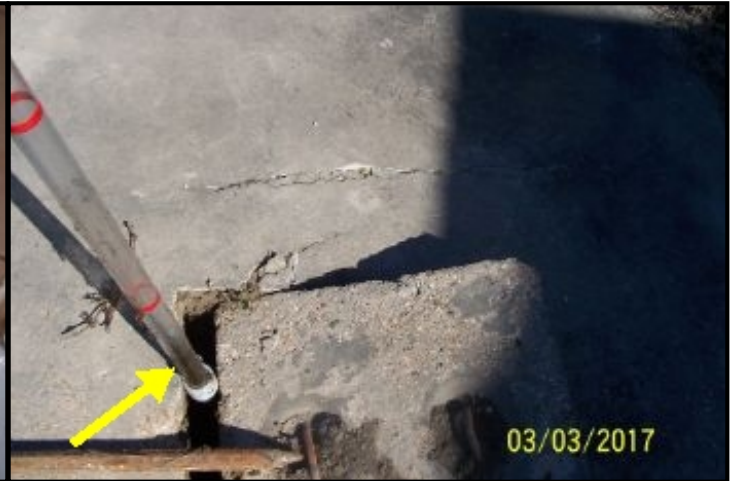
septic tank less than 6" of sludge, no pumping needed at this time
