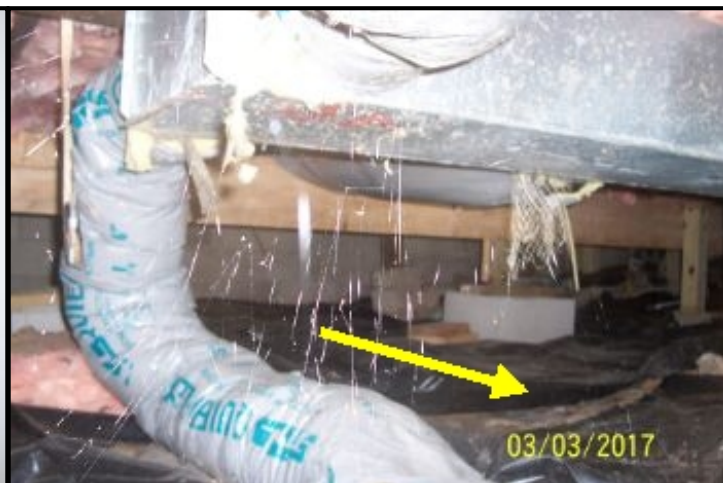
plenum and vent, vapor barrier
