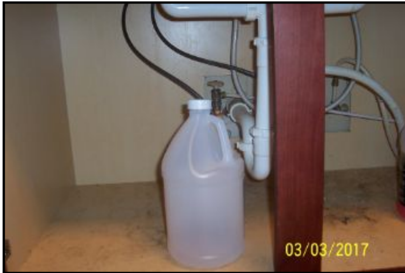
area under sink
