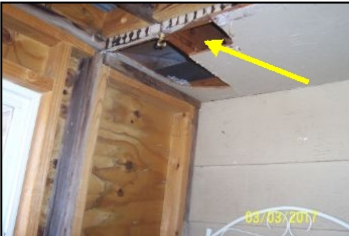
in sun room, not finished
