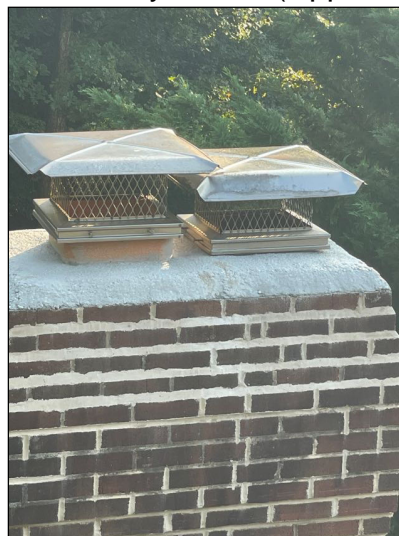
Right Chimney Crown & Cap
