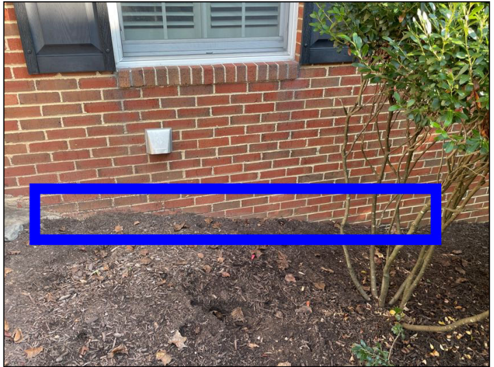
Observed Outdoor Foundation Hidden By Brick
