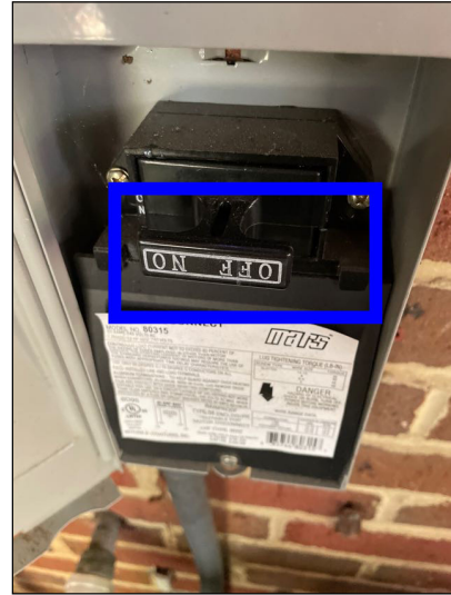
Air Conditioner Electrical Disconnect
