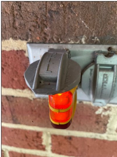
GFCI Outlet Testing Functional
