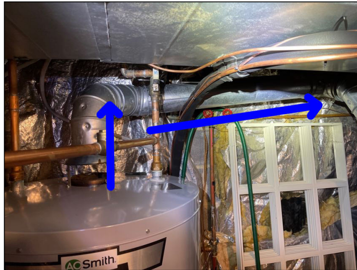
Hot Water Heater Venting Tube
