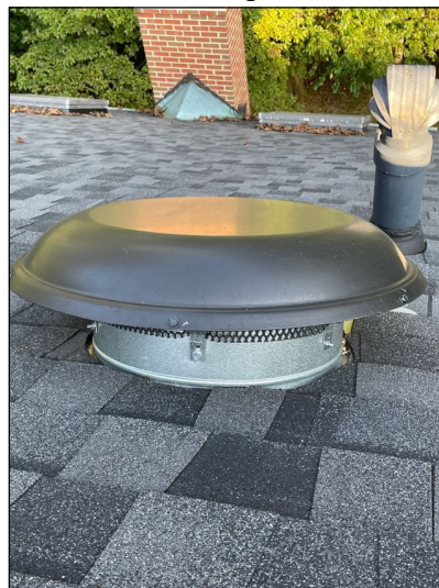
Attic Ventilation Fan (External View)
