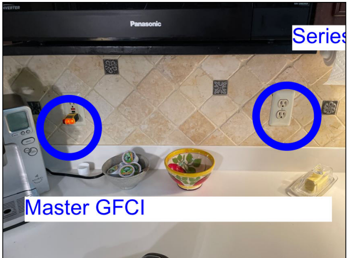
Kitchen GFCI Master (Back Wall)
