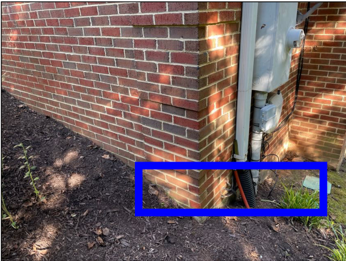
Observed Outdoor Foundation Hidden By Brick
