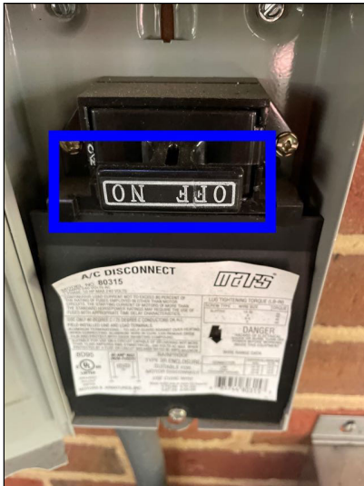
Air Conditioner Electrical Disconnect — Primary Unit
