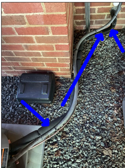
Compressor Refrigerant Line (External)
