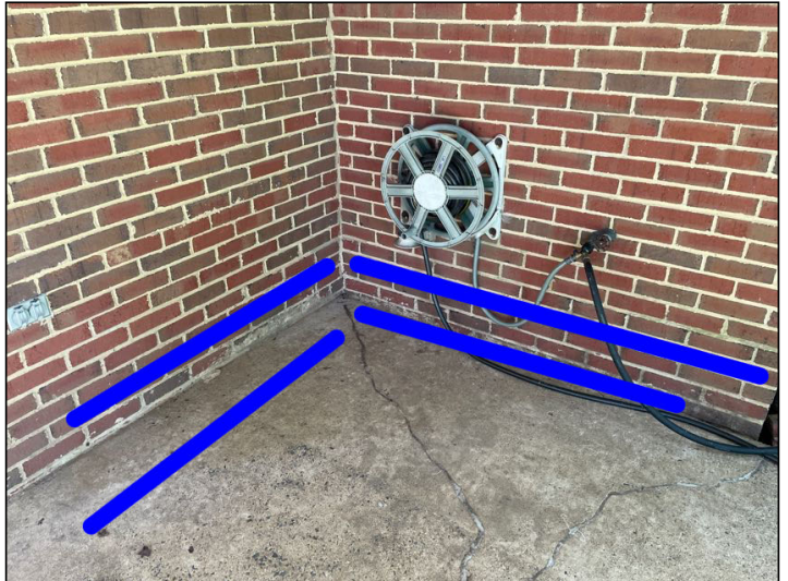
Observed Outdoor Foundation Hidden By Brick
