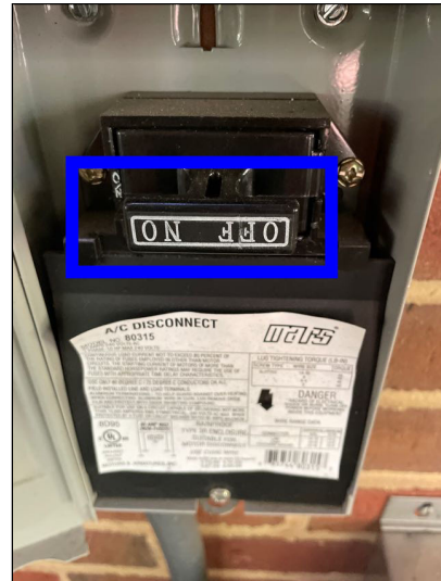
Air Conditioner Electrical Disconnect
