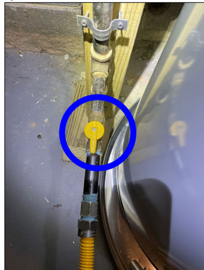
Gas Water Heater Gas Cutoff Noted
