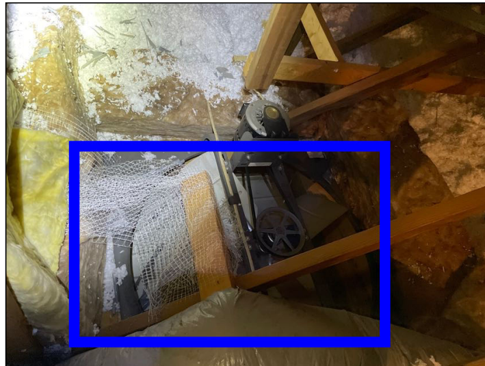
Large 2nd Level Ceiling Fan (Extends Into Attic)
