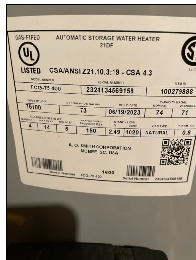
Water Heater Specifications
