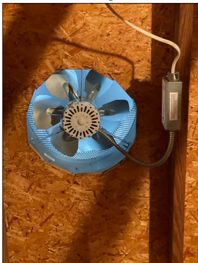
Ventilation Roof Fan (Attic View)
