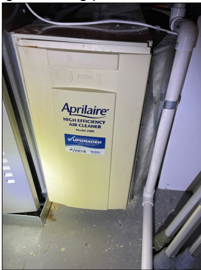
Furnace Filter Housing
