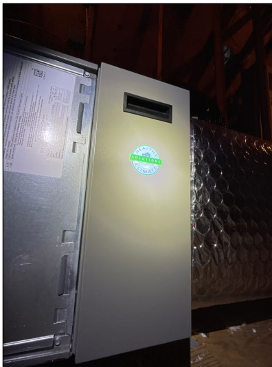
Furnace Filter Housing
