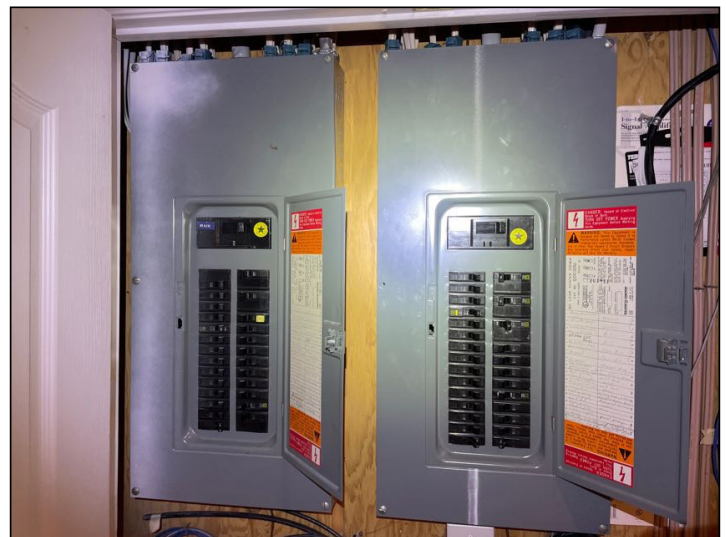
Main Service Electrical Panels -- Covers Open
