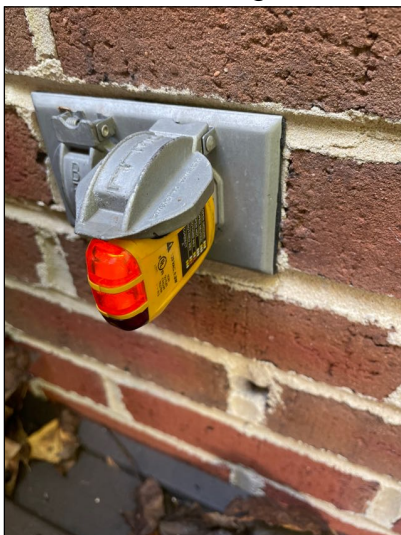
GFCI Outlet Testing Functional
