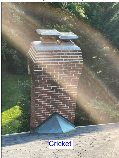
Right Chimney Chase, Crown, Cap & Cricket
