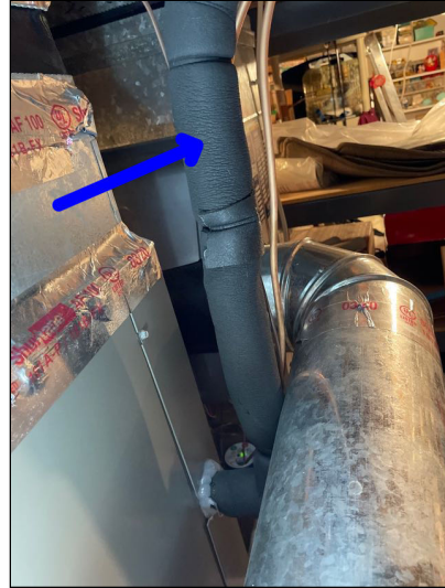
Compressor Refrigerant Line (Internal to Evaporator)
