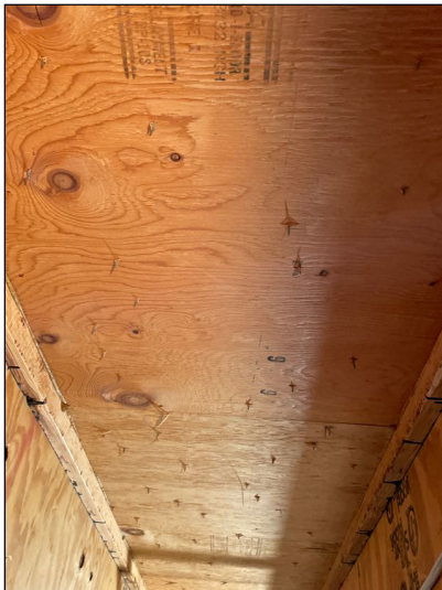
Observable 1st Level Subflooring
