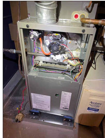
Furnace With Cover Removed
