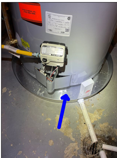
Hot Water Heater Catch Pan
