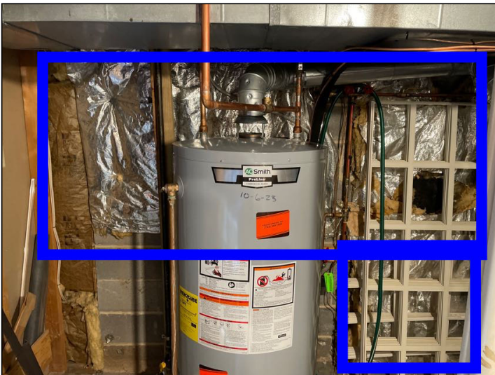
Observed Internal Foundation Area Hidden By Blanket Insulation
