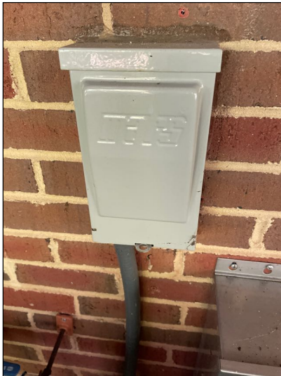
Air Conditioner Electrical Disconnect Box
