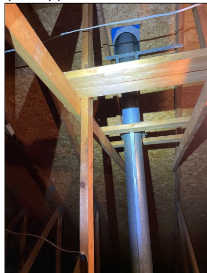
Furnace Venting Tube
