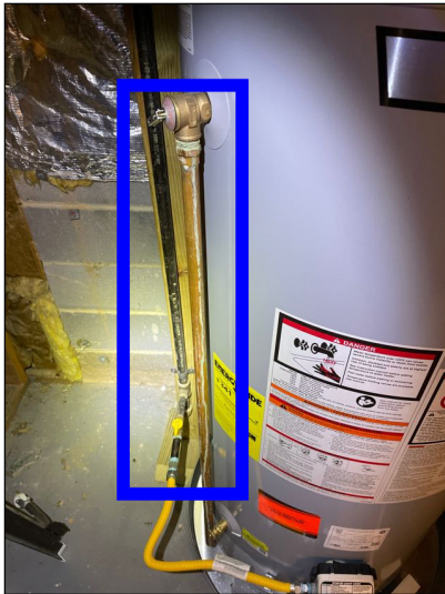
Temperature Pressure Relief Valve
