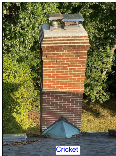
Rear Chimney Chase, Crown, Cap & Cricket
