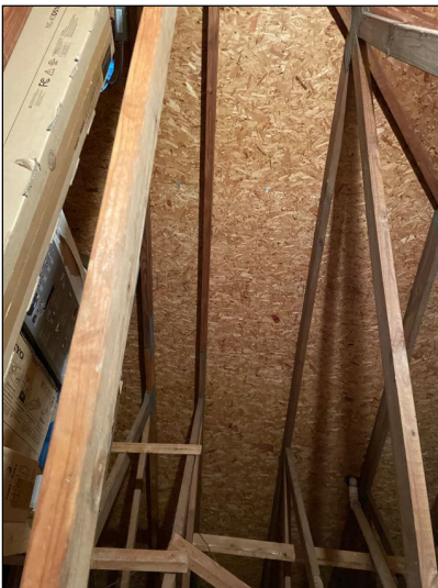
Representative Area of Roof Sheathing
