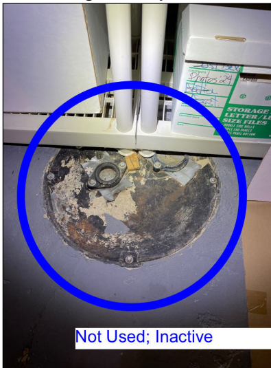
Sump Grinder Pump
