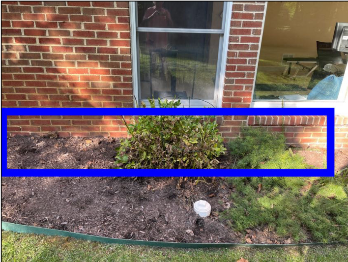
Observed Outdoor Foundation Hidden By Brick
