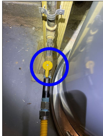
Gas Water Heater Gas Cutoff Valve
