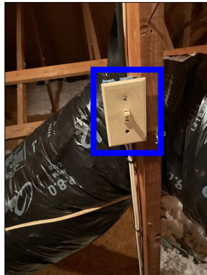
Emergency Shutoff Switch — Unit No 2 (Attic)
