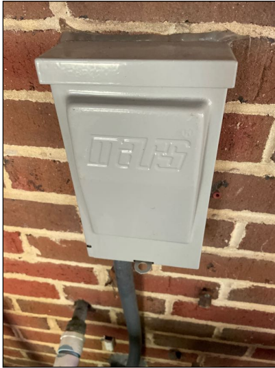
Air Conditioner Electrical Disconnect Box
