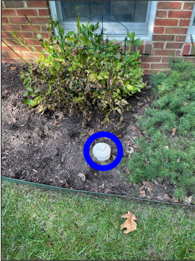
External Plumbing Service Cap
