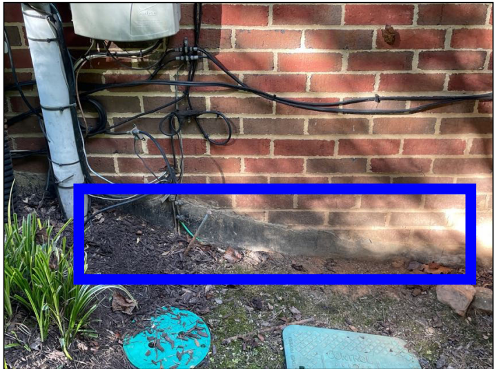
Observed Outdoor Foundation Hidden By Brick
