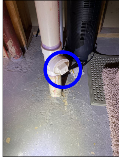
Internal Plumbing Service Cap
