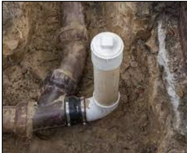
Typical Service Cap For Plumbing Cleanout
