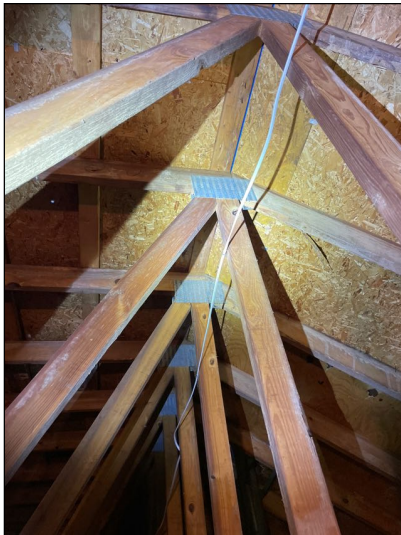
Representative Area of Roof Sheathing
