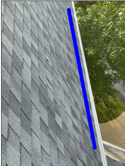
Gutter With Gutter Cap
