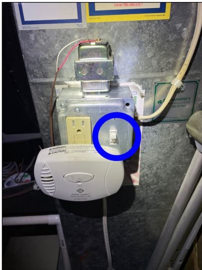
Emergency Shutoff Switch — Primary Unit (Basement)
