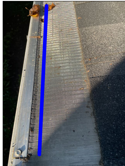
Gutter With Gutter Cap
