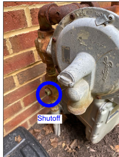
Gas Meter Shutoff Valve
