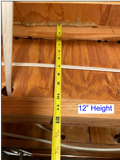
Observable Joists
