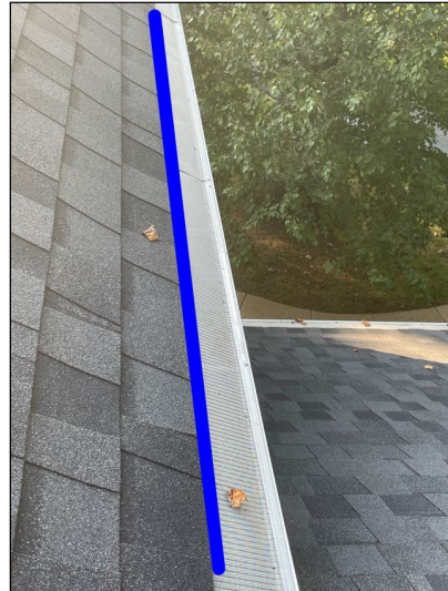
Gutter With Gutter Cap
