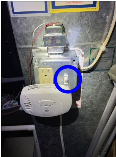
Emergency Shutoff Switch
