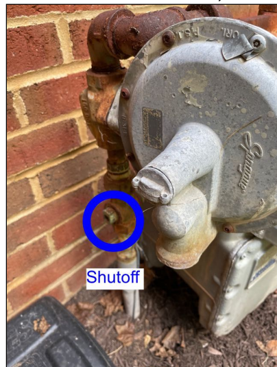
Gas Meter Shutoff Valve
