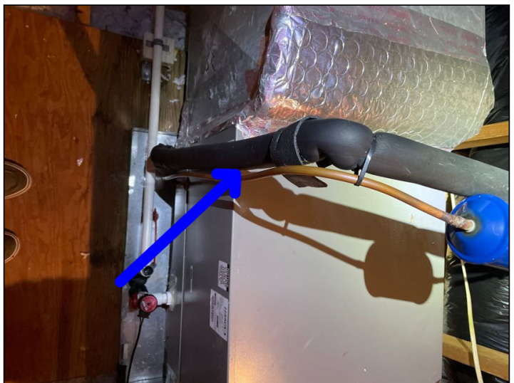
Compressor Refrigerant Line (Internal to Evaporator)
