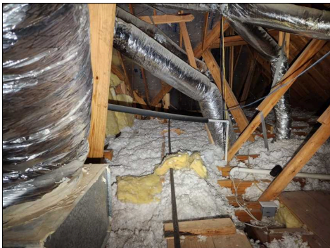
Overview of Main Attic. (Main House)
