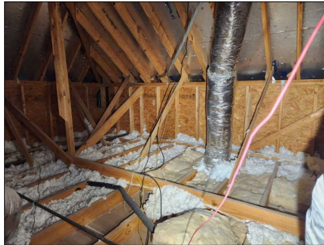
Overview of Attic. Upstairs Right Rear (Main House)
