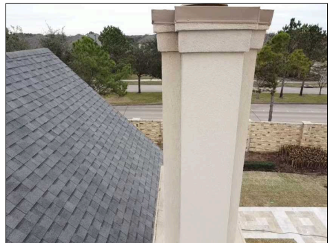
Overview of Living Room Chimney
