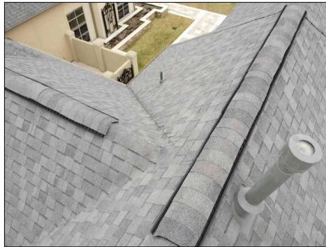
Overview of Roof.
