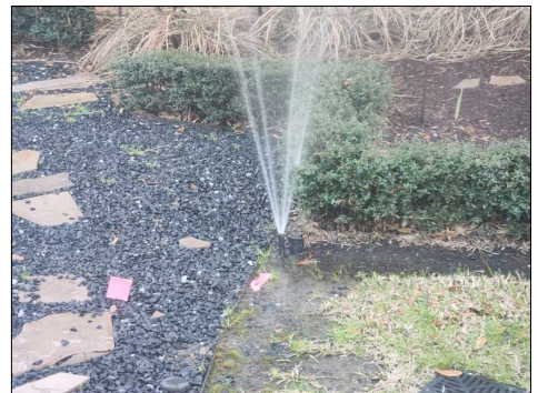
There is a broken sprinkler head. Zone - 12
