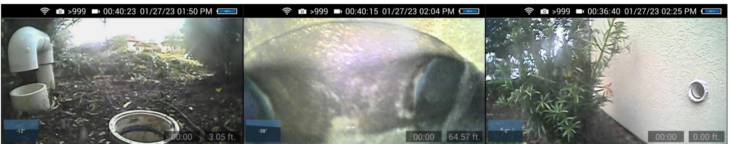
Overview of Sewer Scope Inspection Entry Point (Main House)
