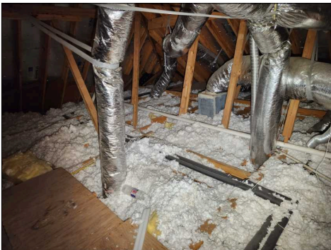
Overview of Main Attic. (Main House)
