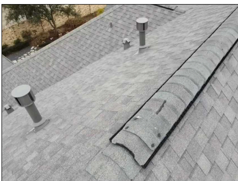
Overview of Roof.
