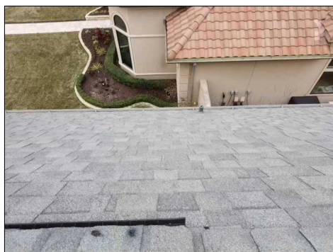
Overview of Roof.
