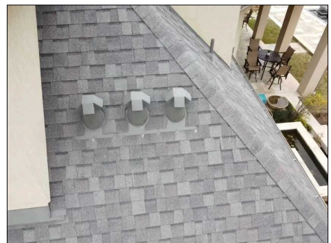
Overview of Roof.
