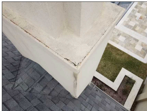
Overview of Living Room Chimney
