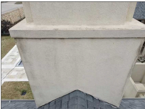
Overview of Living Room Chimney
