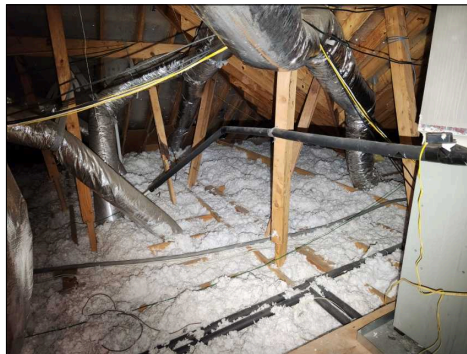
Overview of Main Attic. (Main House)
