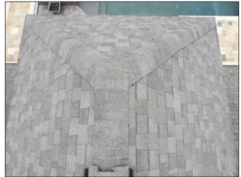
Overview of Roof.
