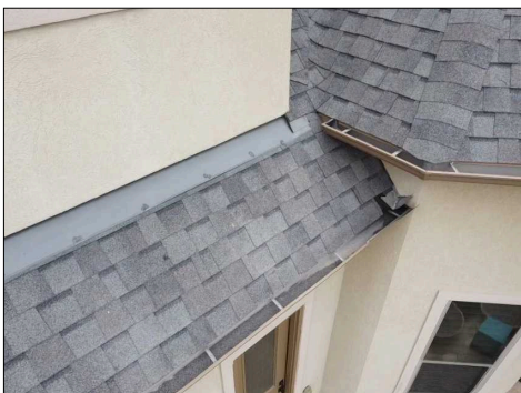
Overview of Roof.
