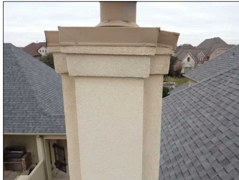
Overview of Living Room Chimney Cap
