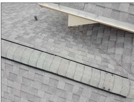
Overview of Roof.
