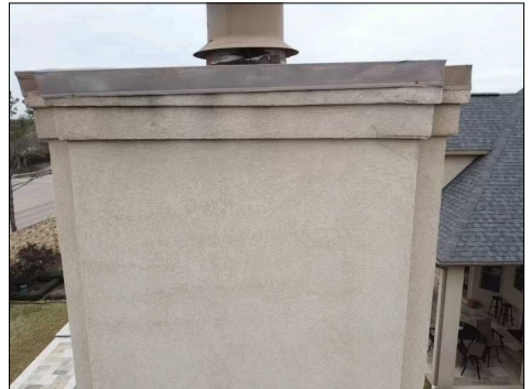
Overview of Living Room Chimney
