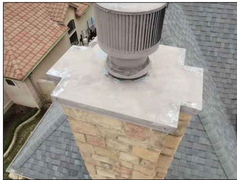
Overview of Office Chimney
