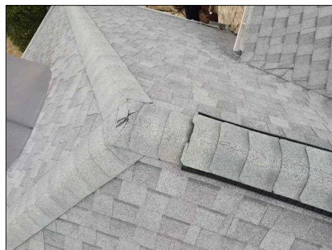
Overview of Roof.
