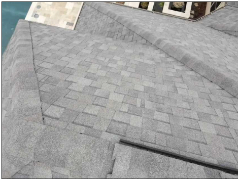
Overview of Roof.
