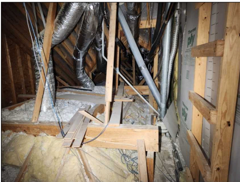
Overview of Attic. Upstairs Left Rear (Main House)
