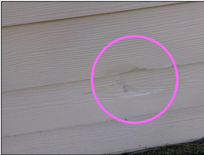
Siding damaged at several locations
