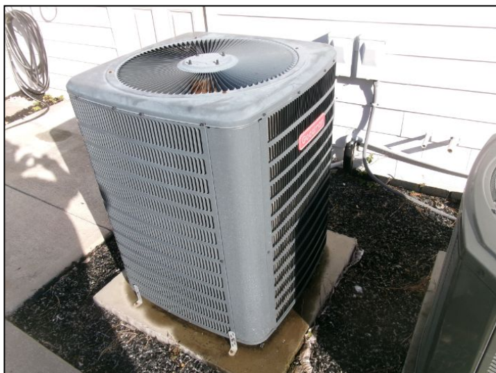
Goodman 2019 03.5 ton electric heat pump (downstairs)
