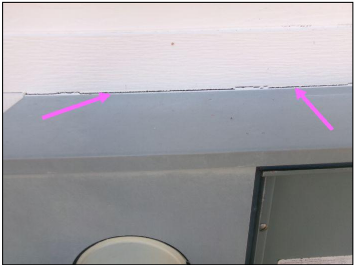
Cracks need sealing
