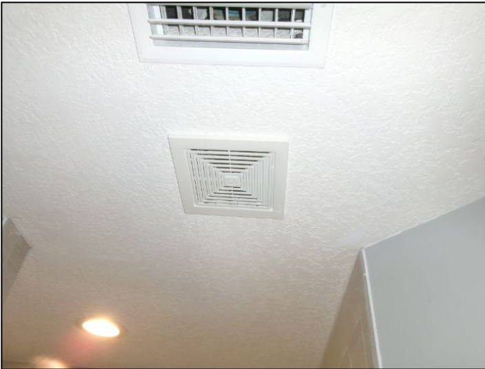
Bathroom exhaust fan inoperative
