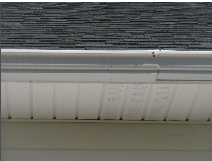
Gutter needs maintenance/repair
