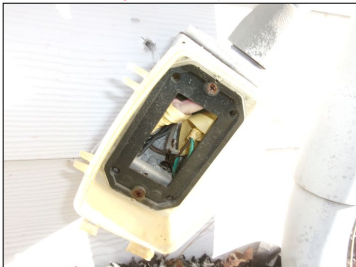
Receptacle damaged
