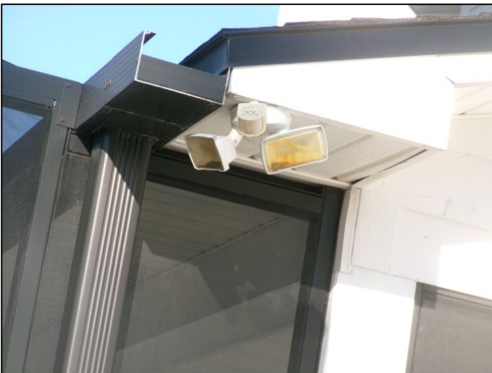
All corner flood lighting is photo cell operated
