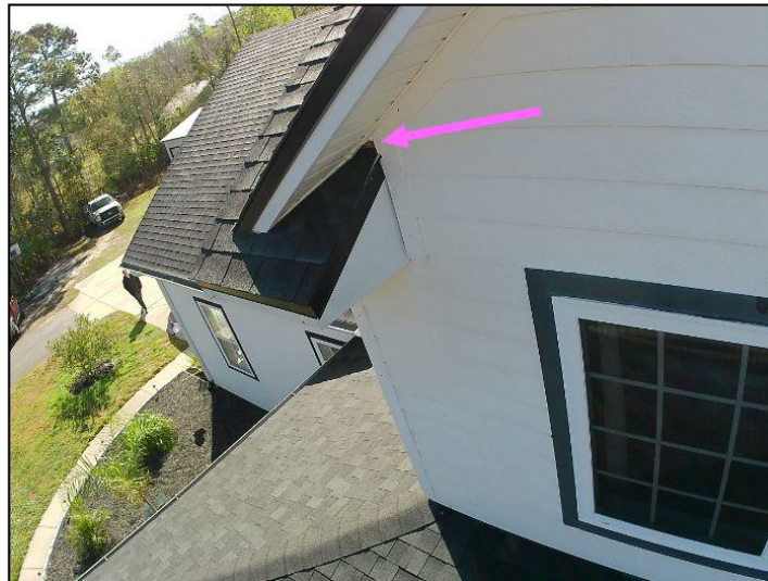
All exterior openings need sealing
