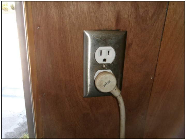
Outlets not GFCI protected
