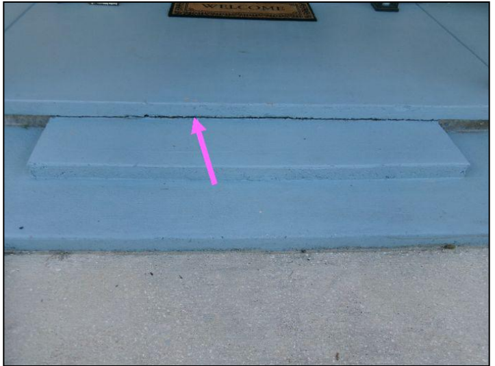
Cracks need sealing
