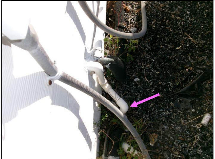
Drain should be moved away from foundation
