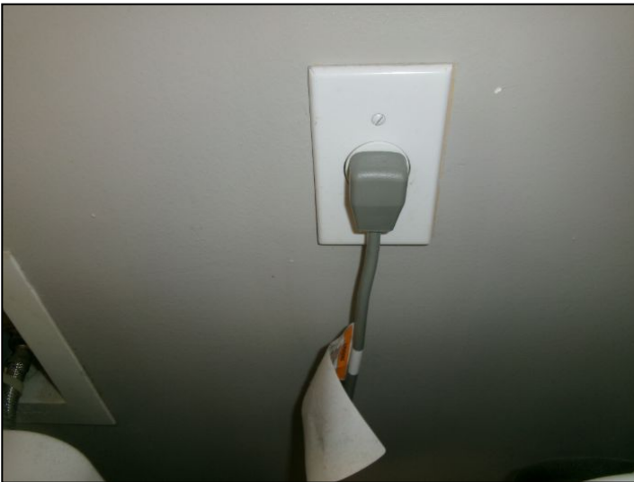
Clothes washer outlet not GFCI protected
