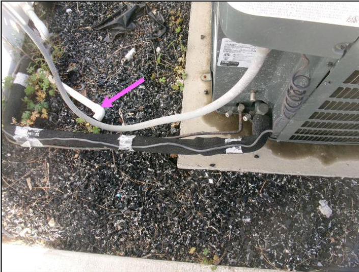
Drain should be moved away from foundation
