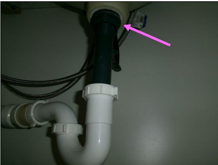
Drain leaks
