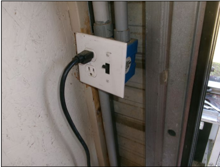
Outlets not GFCI protected
