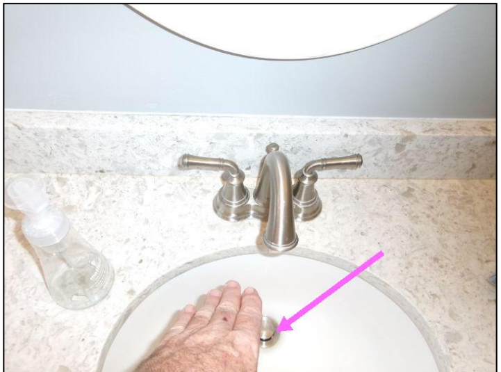
Sink stopper inoperative/missing
