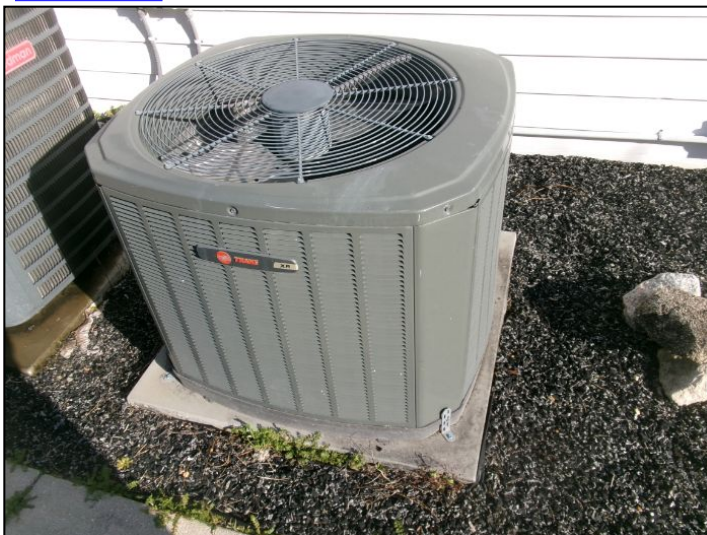
Trane 2019 3 ton electric heat pump (upstairs)
