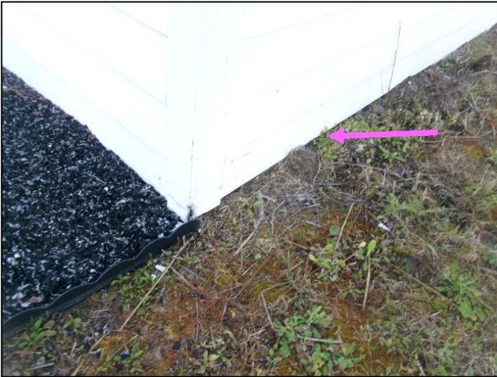
Siding to soil contact
