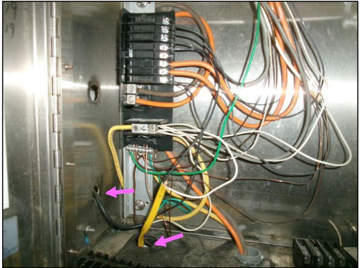
Wires not protected by grommet
