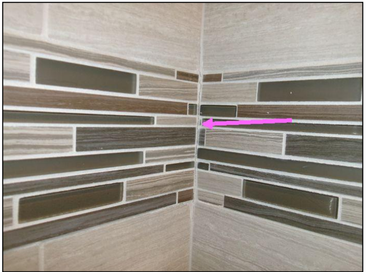
Shower/tub tile needs grout/sealing
