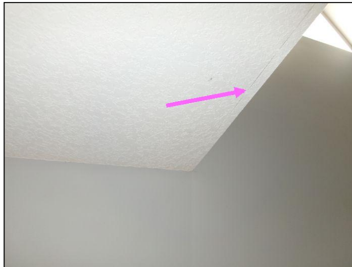
Cracks need sealing
