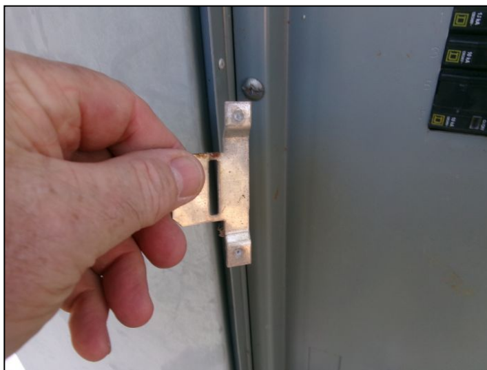
Latch / lock damaged
