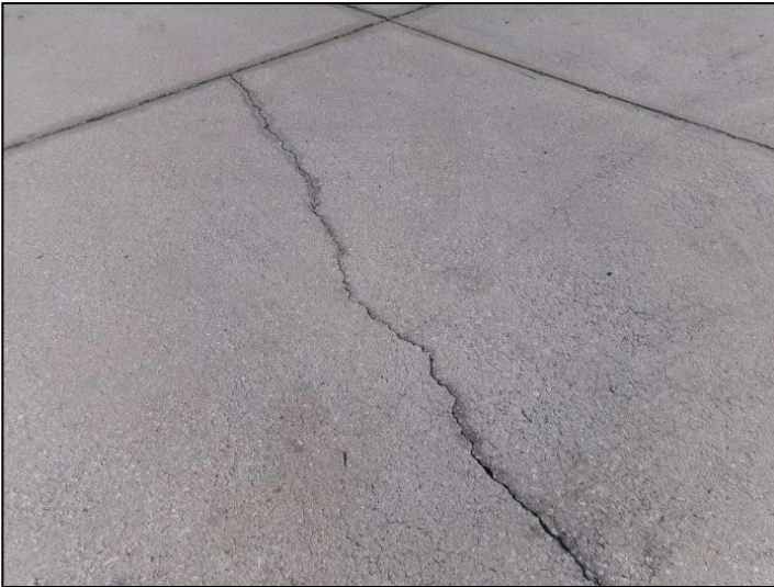
Cracks need sealing
