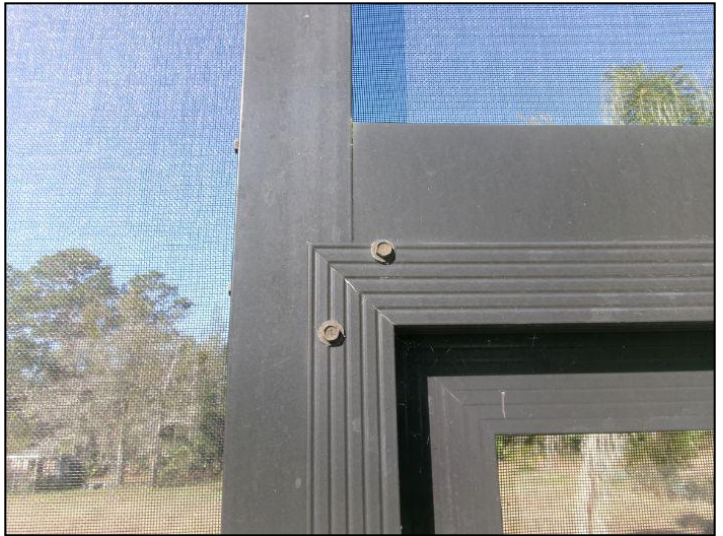
Corrosion on screws
