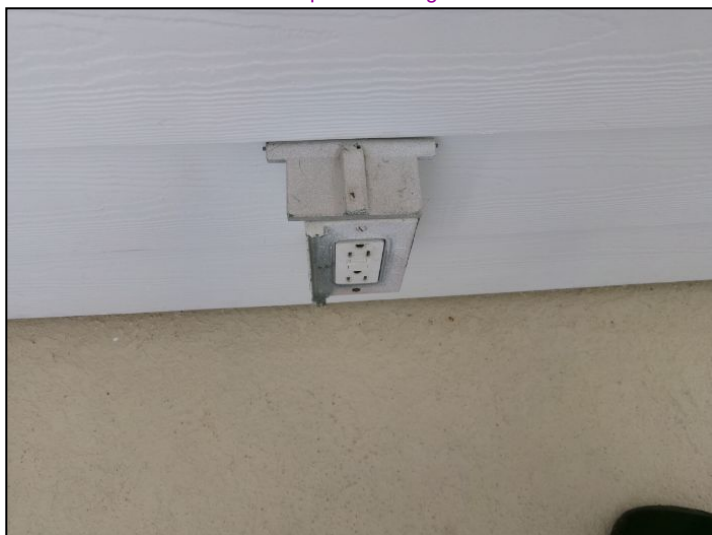
Outlets need weatherproof covers installed
