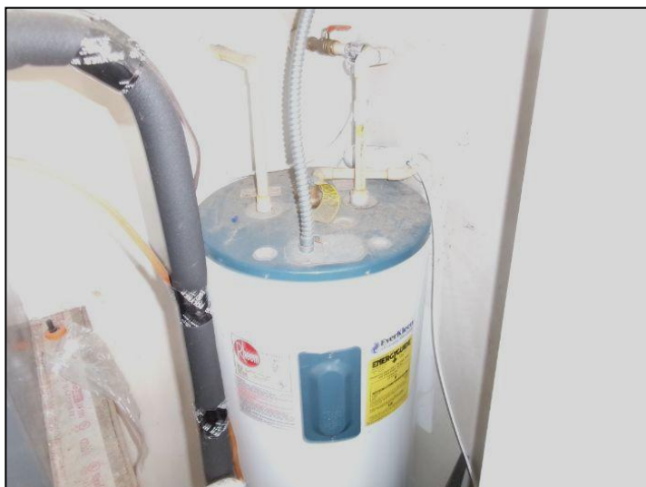
Rheem 2004 40 gallon electric water heater
