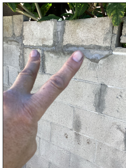
Loose top blocks
